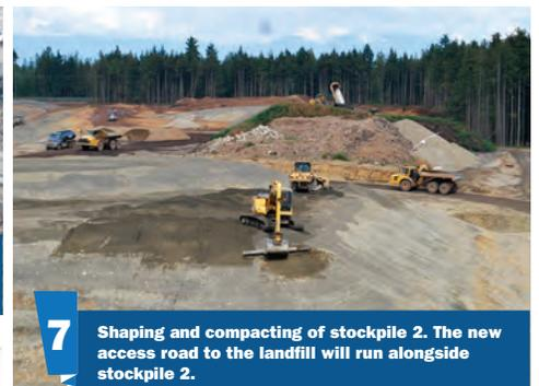
**7** Shaping and compacting of stockpile 2. The new access road to the landfill will run alongside stockpile 2.
